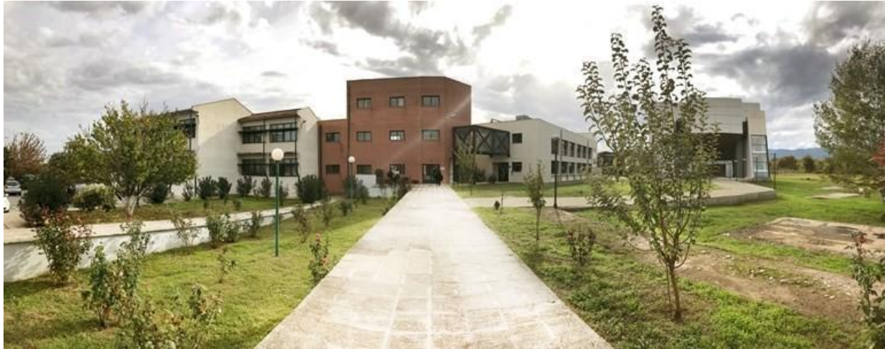
Part of the DPESS facilities.
