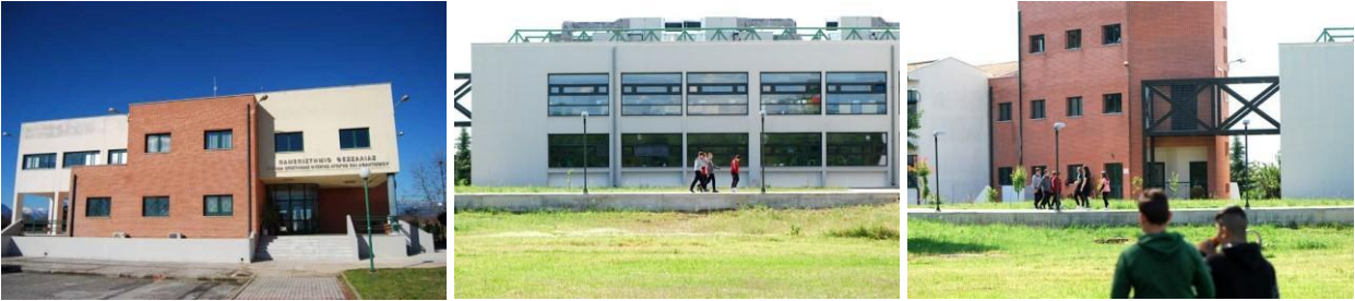
Part of the DPESS facilities.
