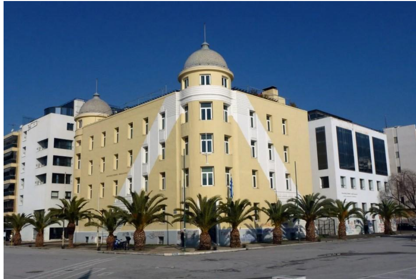
Rector's Building - Administrative Services of the University of Thessaly in Volos (Papastratos Building)
